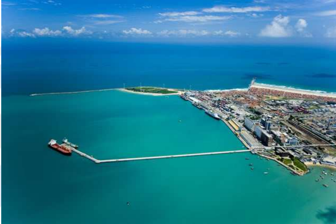
Figure 10 – View of Fortaleza Port (Mucuripe)
